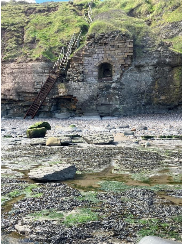
Figure7. Remains of the Cementstone kiln in Hummersea Bay.
