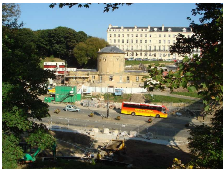
Fig 1. Rotunda Restoration underway in September 2007. Almost complete is the new lower-level entrance and shop area.
